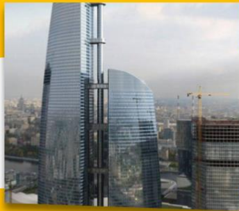
Federation Tower B , Level 62&63 Hyatt Regency Lobby Elektromekanik İşleri
